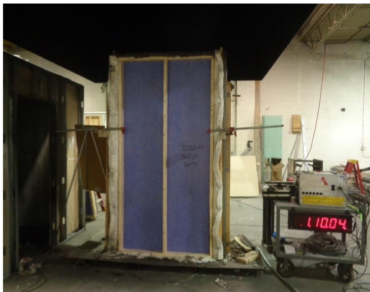
Photo No. 10 Post-test Interior
