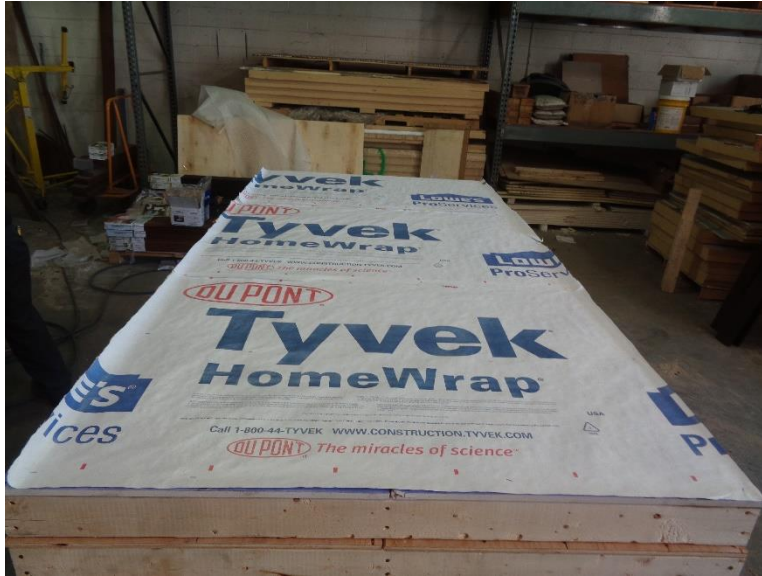
Photo No. 3 Construction of Test Assembly
