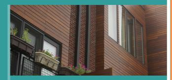
The sustainable alternative to Tropical Hardwood siding. XTR is perfect for architectural designs requiring natural elements on exterior walls. Durable and stable, install with our RainClad<sup>®</sup> Clip Installation System on sheathing or battens.
