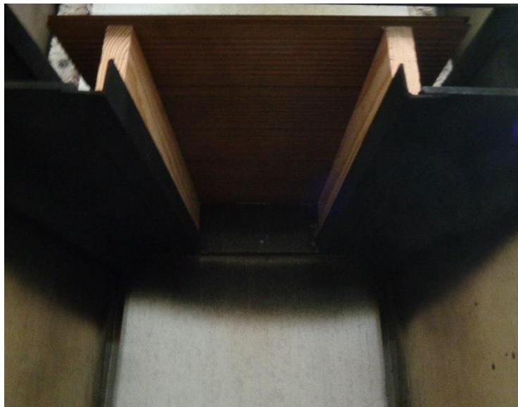
Photo No. 2 Complete Assembly (Below Deck)
