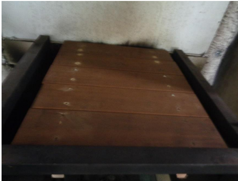
Photo No. 1 Complete Assembly (Above Deck)
