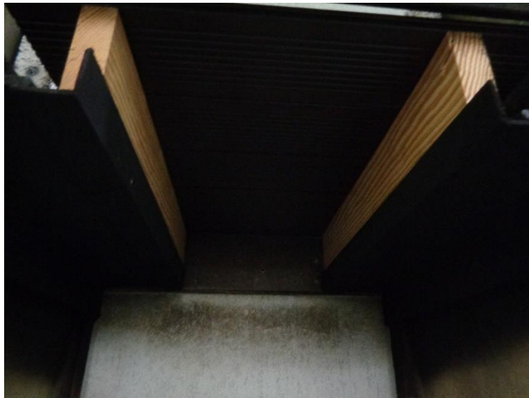
Photo No. 2 Complete Assembly (Below Deck)
